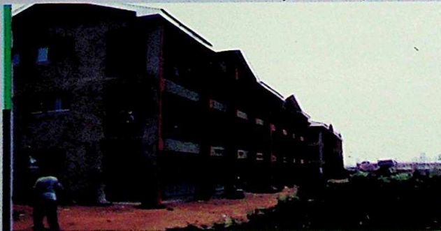
New buildings for the Faculties of Engineering and Biological Sciences, Anambra State University, Uli
