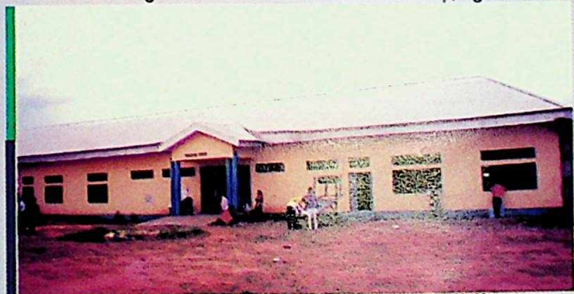
A new Engineering Workshop Building, Anambra State University, Uli
