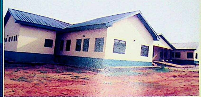
The new Female Ward at Amaku General Hospital
