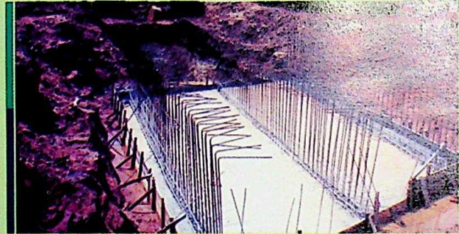
Massive control of erosion at Judges' Quarters, Awka
