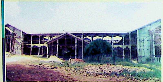
The new Dunukofia Local Government Headquarters under construction
