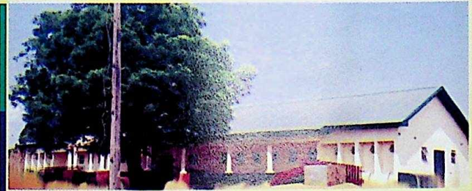
Another new structure at Umueri General Hospital
