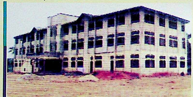
Main building of Awka North Secretariat, which construction is nearing completion
