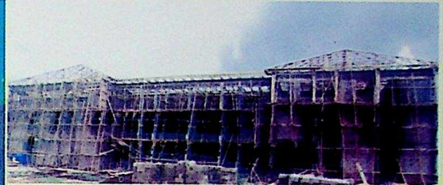
Consultants Clinic under construction at Amaku General Hospital
