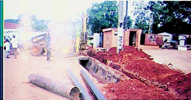
The laying of pipes for Amawbia Water Scheme
