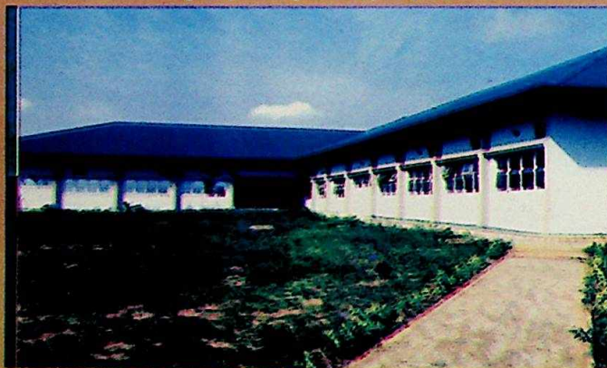
State Emergency Management Agency's new office building, which has an Emergency Unit
