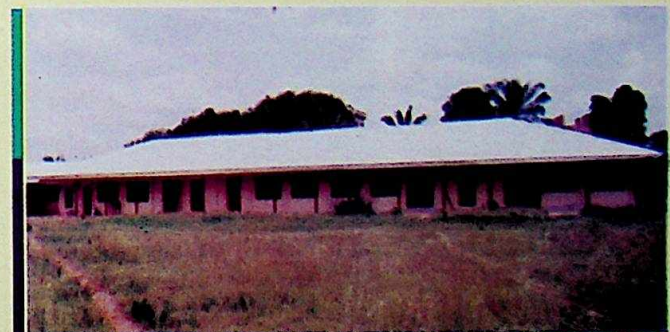
A new Classroom Block at the College of Health Technology, Obosi
