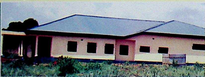
Yet another new structure at Umueri General Hospital
