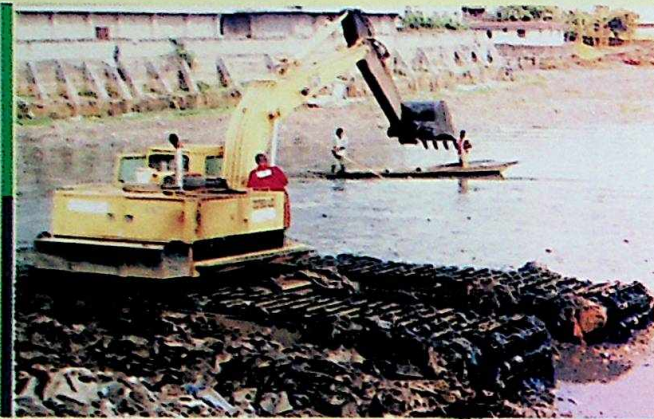
The dredging of Nwangene Creek, Onitsha the first since Independence. The creek has wreaked havoc in the area over the years
