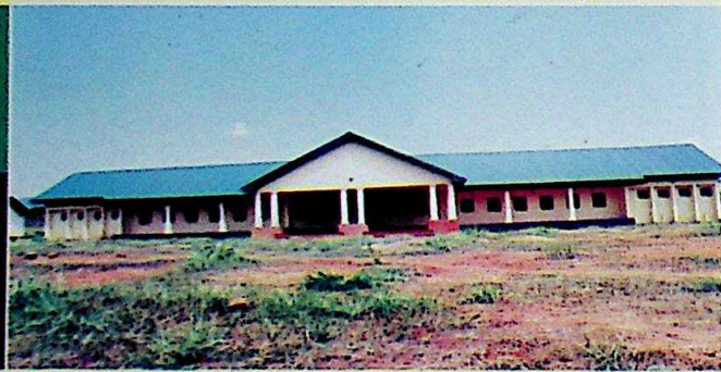
Umueri General Hospital, re-built from foundation by Governor Peter Obi, after it was burnt down completely during the communal disturbances in the area in 1995
