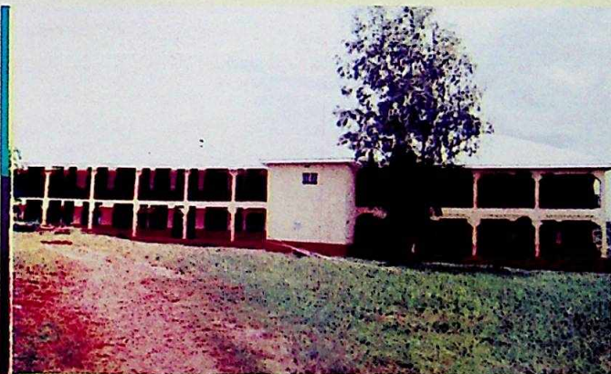
A new Auditorium at the School of Nursing, Nkpor, which has been accredited
