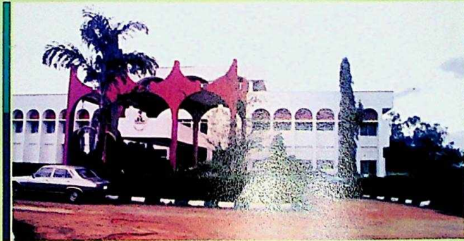
The State House of Assembly Complex, rehabilitated and furnished by Governor Peter Obi
