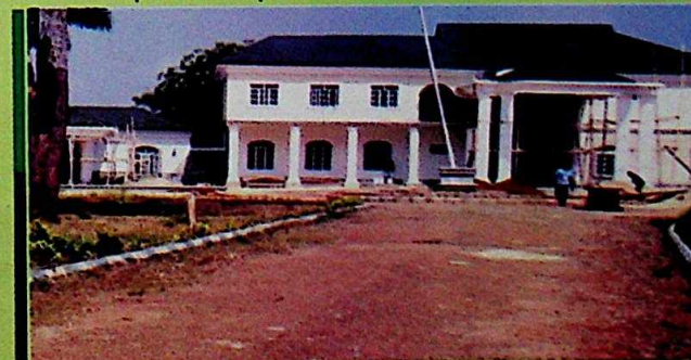
The new Governor's Lodge, Onitsha built by Governor Obi
