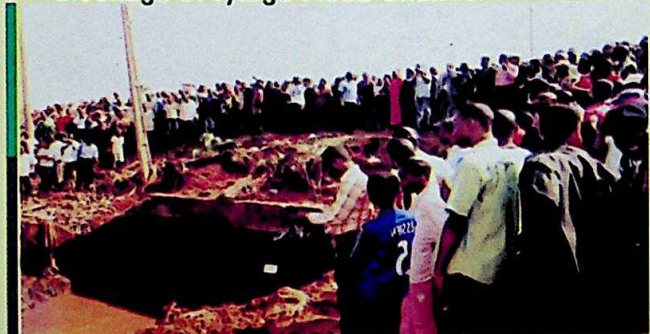
Opening up of the Iyiagu Flood Channel in Awka, blocked for 10 years under previous Administrations, with untold hardship to the people
