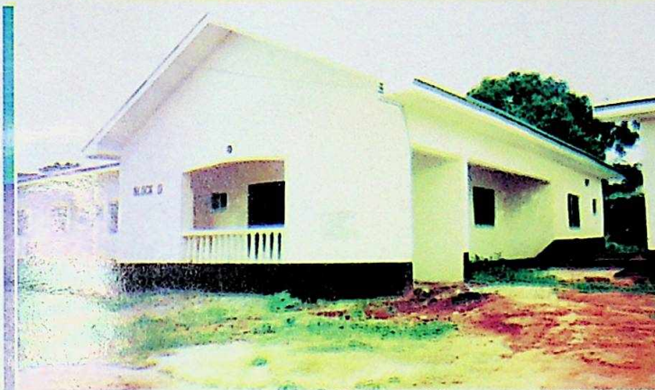
A new block of Resident Doctors' Quarters, built by Governor Obi at the Onitsha General Hospital
