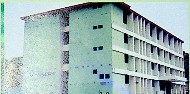
Ministry of Justice Building, Onitsha. The State has similar buildings at Newui, Otuocha and Ekwulobia
