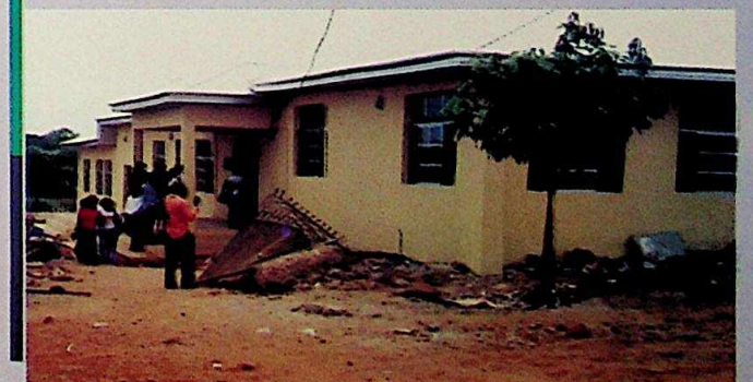
A new classroom building at Anambra State University, Igbariam Campus
