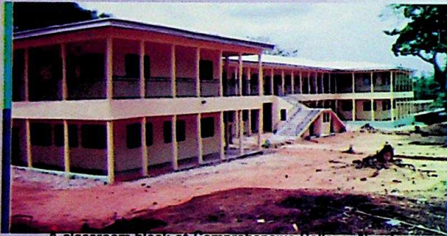
A classroom block at Comprehensive College, Nawfia; another collaborative effort between Government and corporate organizations
