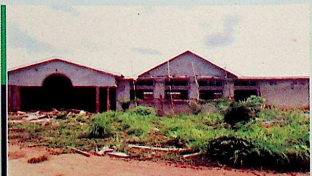
A classroom block at the College of Agriculture, Mgbakwu
