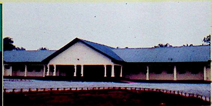
Another new structure completed at Umunze Cottage Hospital
