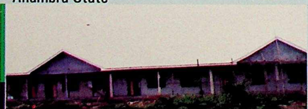
Since the College of Agriculture was relocated from Igbariam to Mgbakwu, no former Governor built even a hut there, but Governor Obi has built eight structures including this Hostel Block
