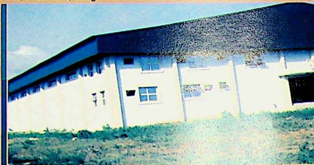
A new store building for the State Emergency Management Agency
