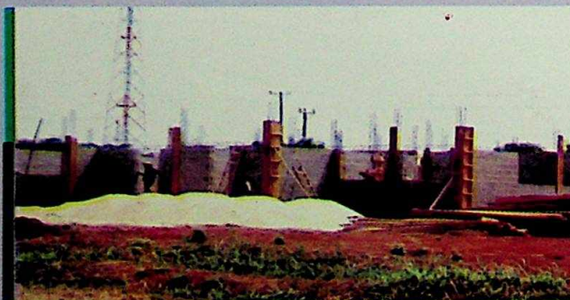
A building under construction at Nwafor Orizu College of Education, Nsugbe
