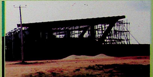
Amphitheatre at the Women's Development Centre, Awka, under construction
