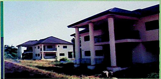
Two of the many buildings at Judges' Quarters, Onitsha, the first ever in the State
