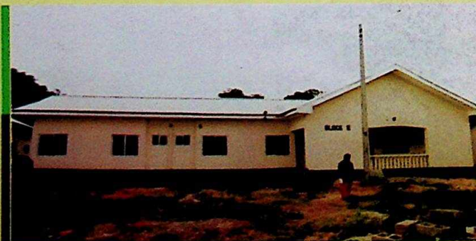
Another new block of Resident Doctors' Quarters, Onitsha General Hospital
