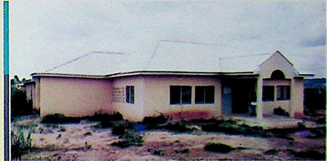
A new Hostel Block at the School of Midwifery, Nkpor
