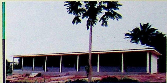
A new Classroom Block at the School of Midwifery, Nkpor
