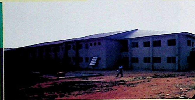
A new 200-bed hostel at the School of Health Technology, Obosi
