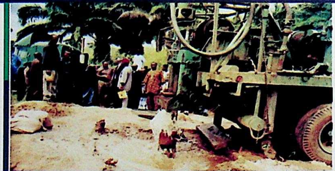
The Enugu Agidi Water Project for Awka Water Scheme
