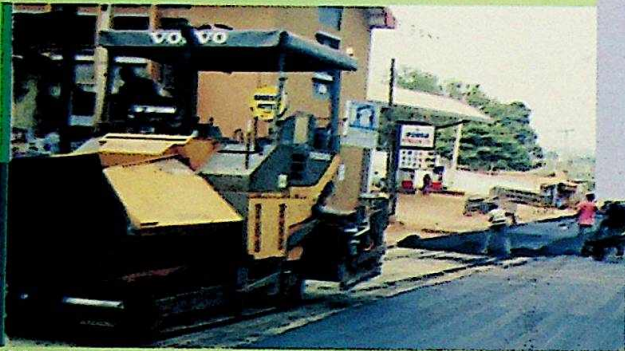
Massive construction of roads going on in the State
