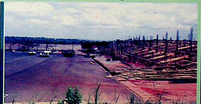
Pavilions being erected at Ekwueme Square, Awka
