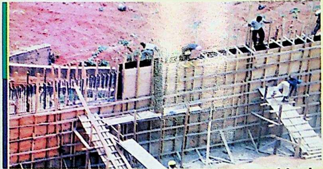
The on-going control work in Umuchiani Erosion Site, Ekwulobia
