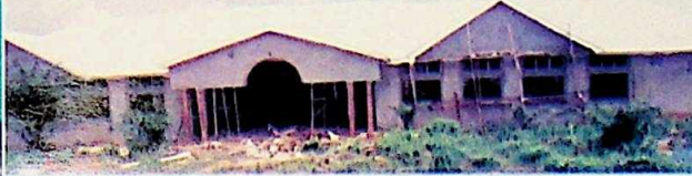
A Classroom Block at the College of Agriculture, Mgbakwu
