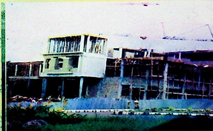
Phase II of the State Secretariat, Awka (on-going)
