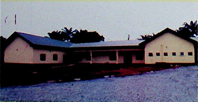
A new structure completed at Umunze Cottage Hospital
