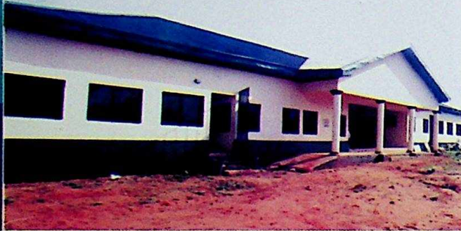
The new Male Ward at Amaku General Hospital, Awka
